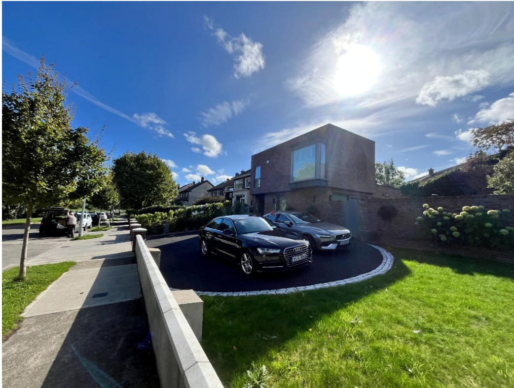
Figure B2. No. 39A Finsbury Park. Contemporary flat-roofed form, projecting upper volume and corner glazing, seen alongside the neighbouring pitched-roof houses.
