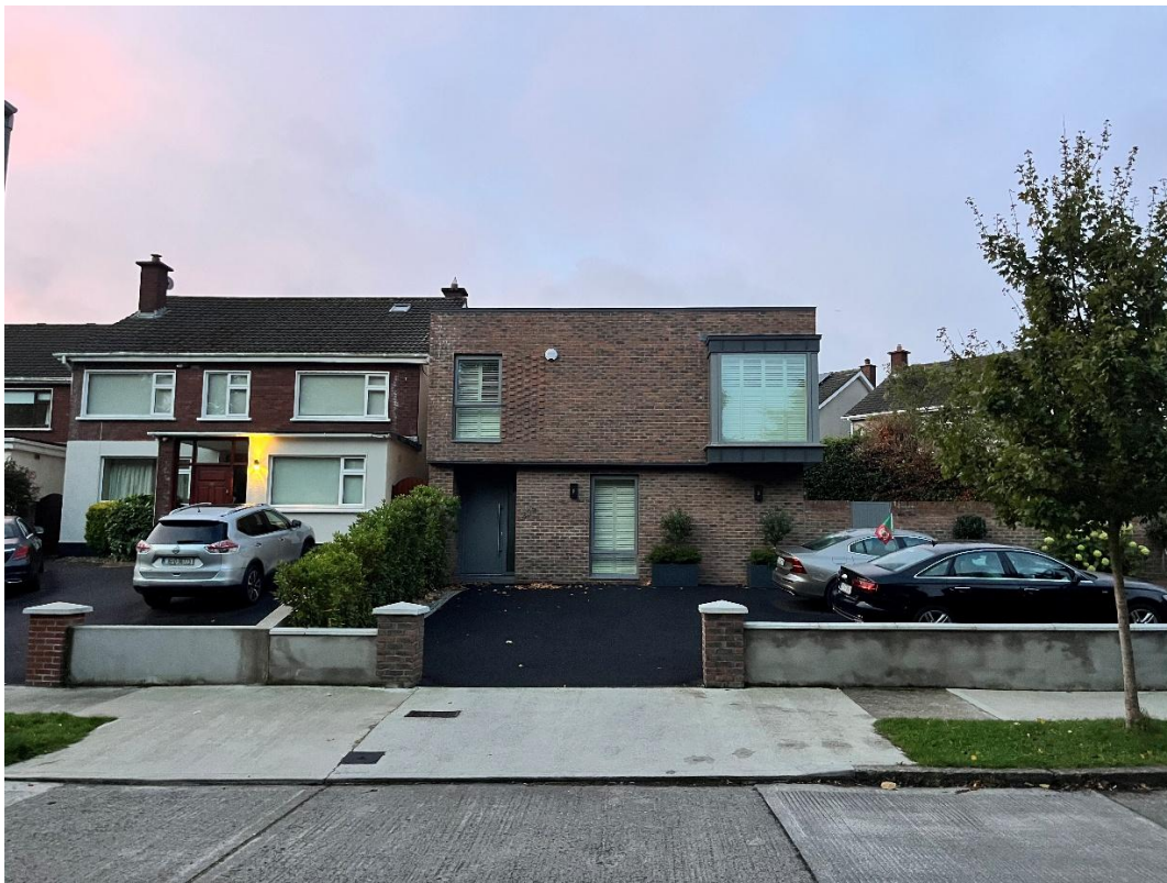
Figure B3. No. 39A Finsbury Park viewed from the front, showing its contemporary flat-roofed form, asymmetric fenestration and projecting upper-floor glazing beside the adjoining pitched-roof dwelling. The view illustrates the contrasting roof forms and façade compositions accommodated within the same streetscape.
