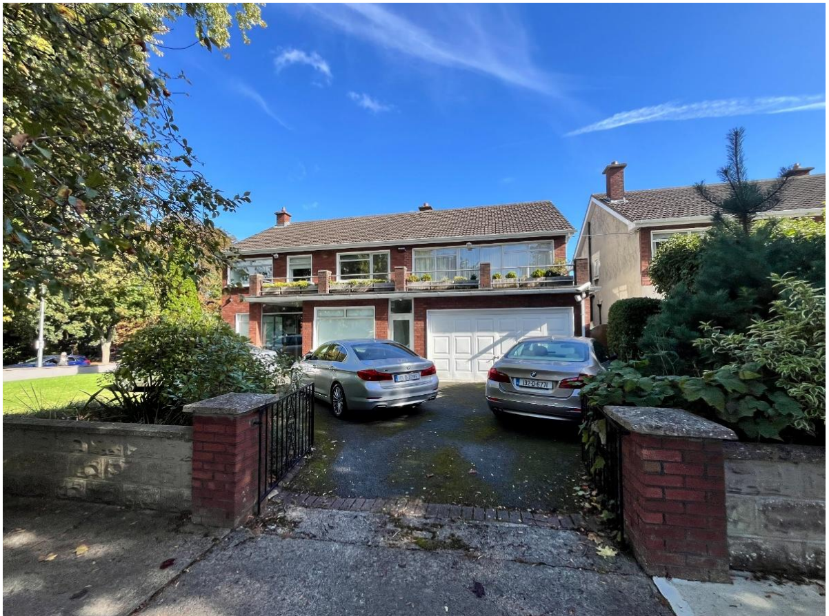
Figure B1. No. 38 Finsbury Park. The broad front elevation, long first-floor balcony, extensive glazing and garage frontage provide a distinctive composition within the estate.
