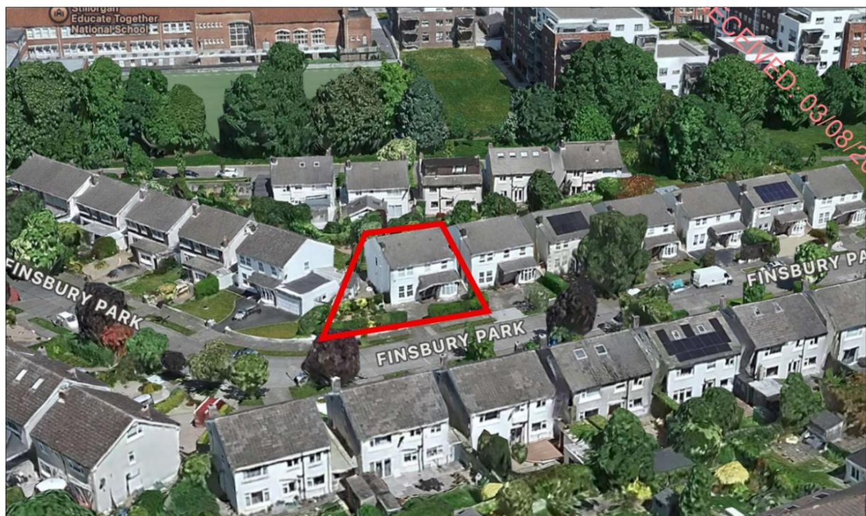
Figure A2. Aerial view showing No. 33, outlined red, at the bend in the road and its relationship with adjoining houses. Reproduced from Figure 2 of the Planning Statement. Original source: Google Maps.
